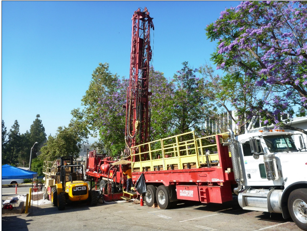
Figure 3-1. Pilot Hole Drilling
