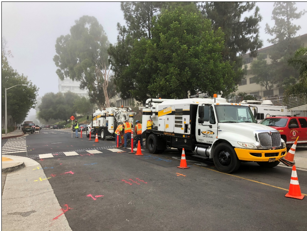
Figure 5-1. Air Knife Trenching on Explorer Road
