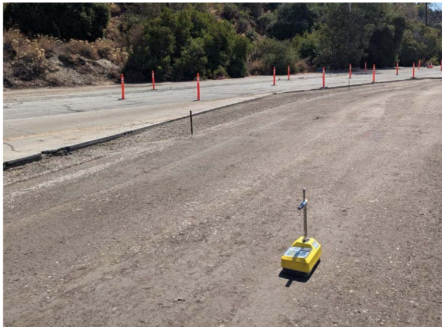
Image 1: Taking nuke gauge density reading on base layer at test location #4.
