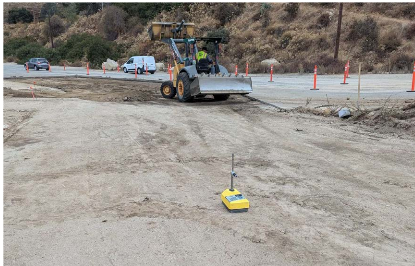
Image 1: Taking nuke gauge density reading on subgrade at test location #3.
