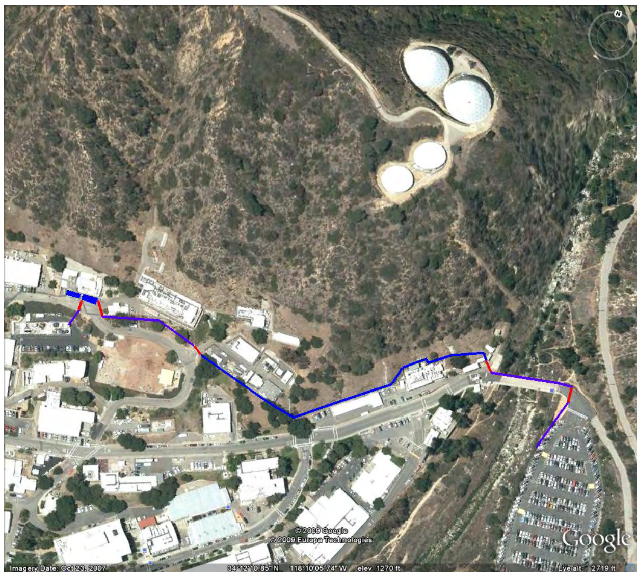
Overview of Pipeline Run on JPL Facility
